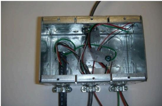
**Fig. 3-4 Rough plumbing and wiring to rough-in box, flush mount unit**
